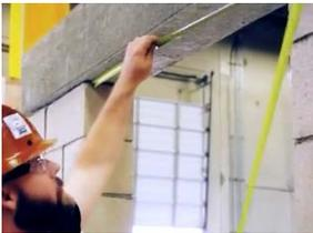
**Note:** the rough opening shall be no less than  $\frac{1}{4}$ " larger in width and  $\frac{3}{16}$ " in height than the frame. The maximum rough opening should not exceed  $\frac{3}{8}$ " larger than the frame width and  $\frac{1}{4}$ " in height.
