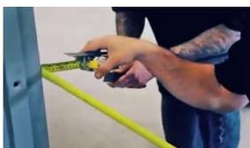
10. Add shims to the jambs and measure to ensure the appropriate width is maintained. Align the hinge jamb to the chalk line. Check the jamb for level and plumb.
