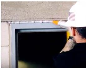
15. Remove the string and spreader bar. Fill any gaps between the frame and wall with caulk or a backer rod. Your frame installation is complete and is now ready for the next phase of construction.
