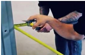
14. Begin anchoring the strike jamb in the same sequence as the hinge jamb. Be sure to check the width at the center of the frame as you install the anchors.
