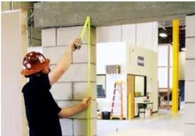
2. Ensure the rough opening has the proper dimensions per the manufacturer's installation instructions. Be sure to check the opening height in two places across the width of the opening. The width should be measured at three places – top, middle, and bottom. This will help you determine the amount of shimming that may be needed to install the frame.
