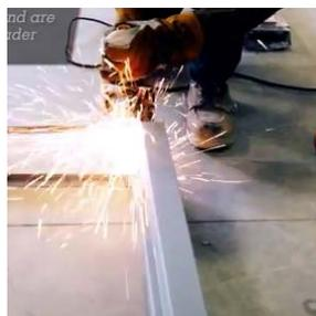
5. If you are installing a welded frame, remove the shipping spreader bar before placing the frame in the opening.
