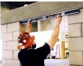
3. Check the opening for plumb, level, and square. Use a 6' level for both jambs and a framing square for the corners. If the rough opening is out of spec for plumb, level or square, do not proceed with installing the frame.
